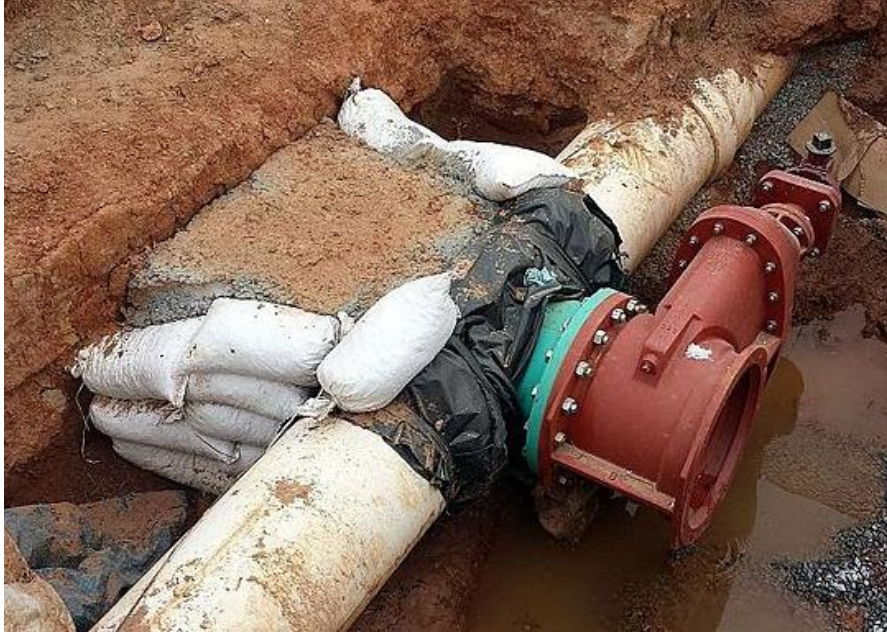
Figure 6.14: An exposed flanged joint 54
