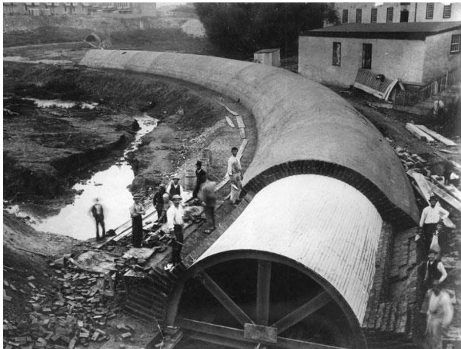
Figure 1.7: Mill Creek Sewer 7
