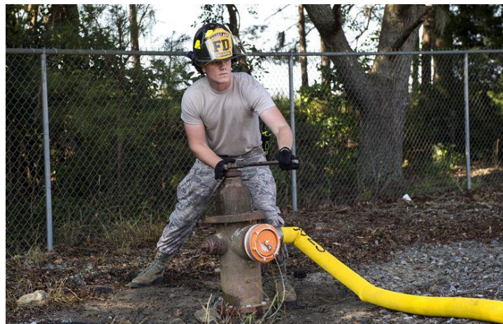
Figure 8.7: Closing a fire hydrant bonnet 84
