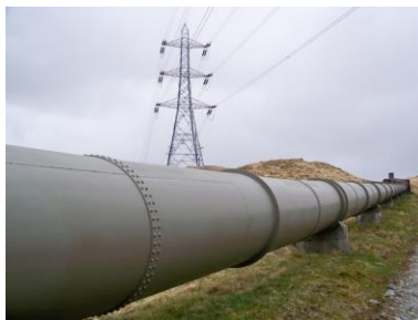
Figure 6.1: A transmission water main 40
