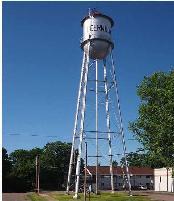
Figure 5.2: Elevated metal water tower 37
