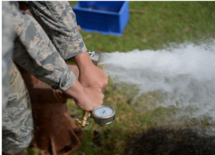
Figure 4.4: Fire hydrant repair 30
