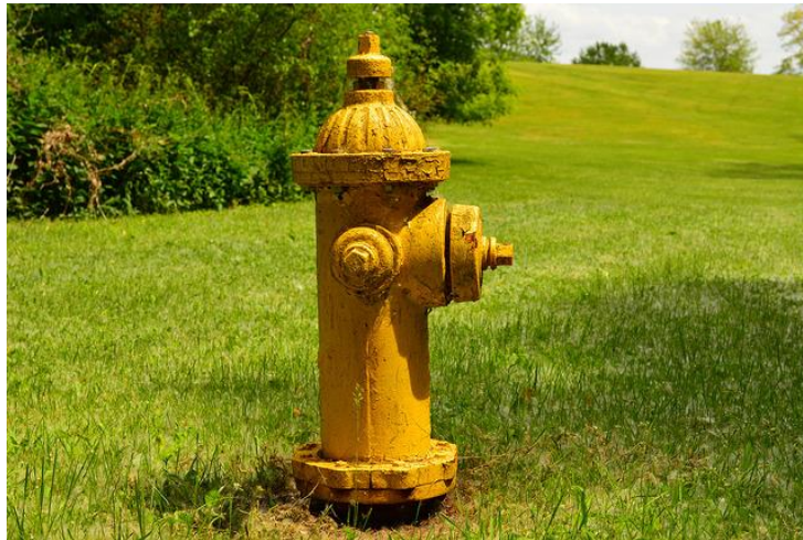
Figure 8.3: A yellow fire hydrant 80
