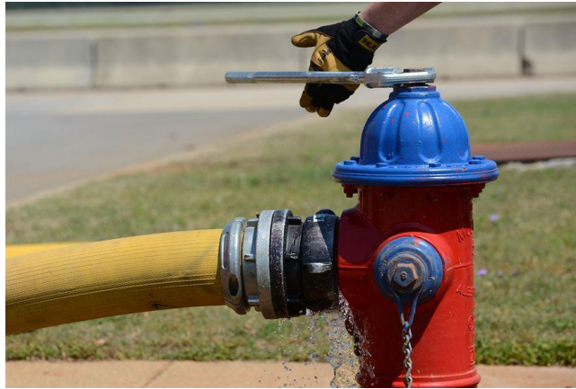
Figure 8.5: Pumping water out from a fire hydrant 82
