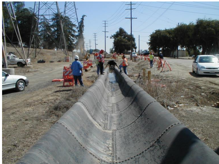
Figure 6.7: Steel pipe maintenance 46
