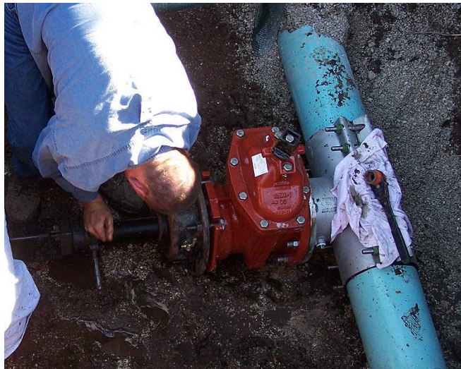
Figure 7.9: Municipal gate valve repair 65
