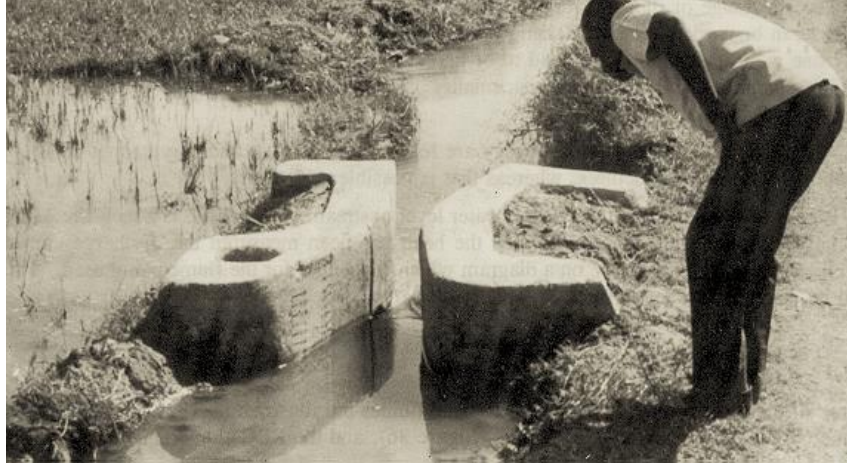
Figure 9.6: A flume mechanism 94
