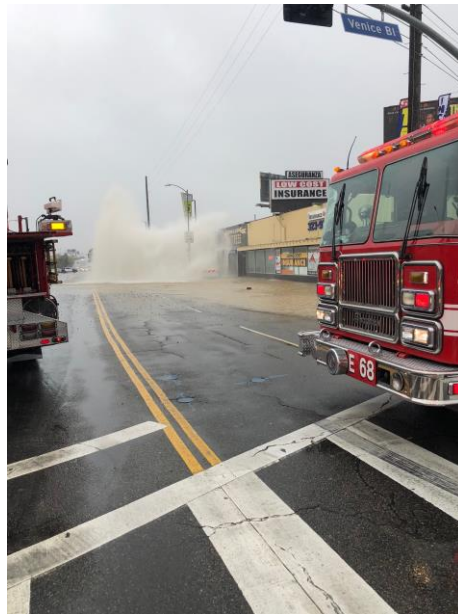
Figure 1.9: The Los Angeles Fire Department responding to a damaged pipe 9
