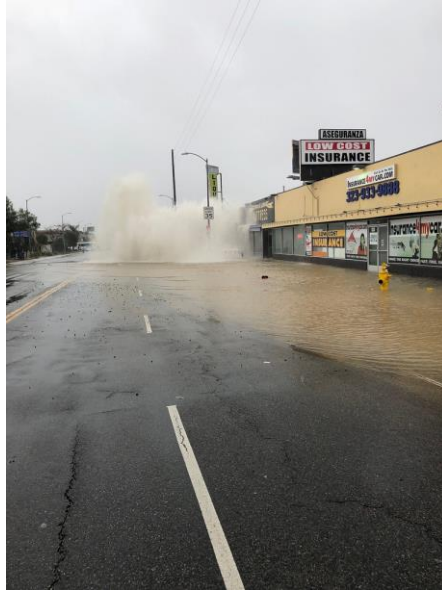
Figure 4.8: A pipe rupture in Los Angeles 34
