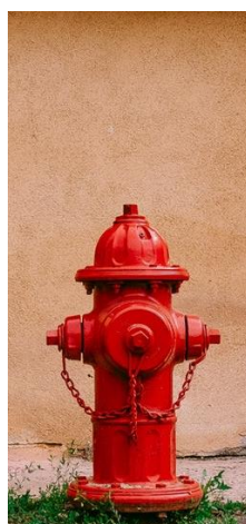
Figure 8.1: A fire hydrant 78
