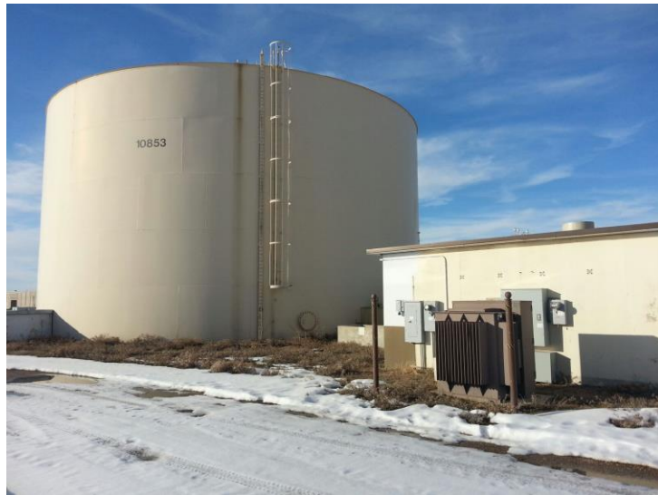
Figure 5.4: An above ground storage tank 39
