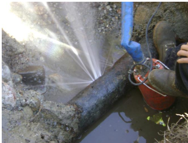
Figure 4.9: A pipe leak repair 35
