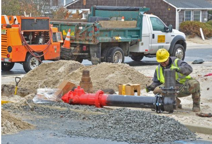
Figure 8.8: A workman installs a new fire hydrant 85
