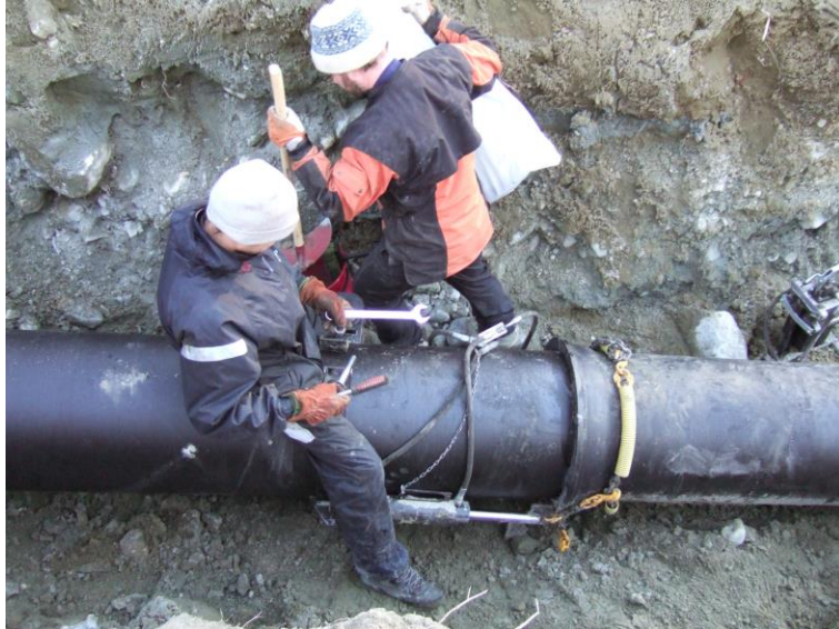
Figure 6.6: The maintenance of a ductile iron pipe 45
